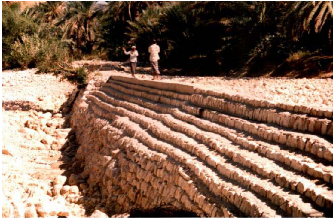
Figure 7 Qaid with stairs
